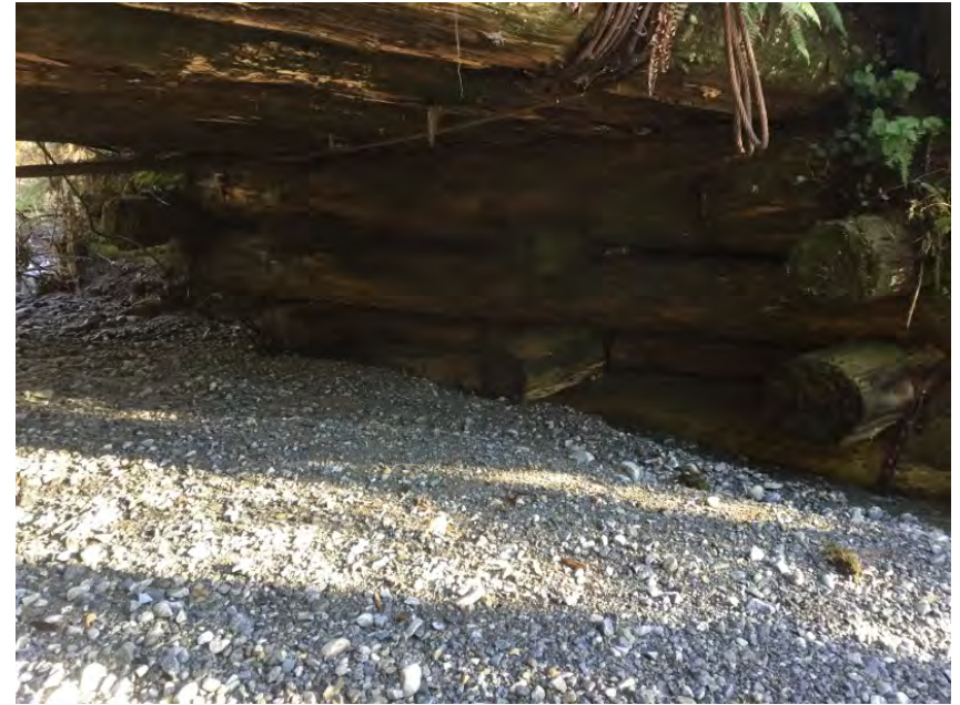
Left Bank Abutment when facing downstream
