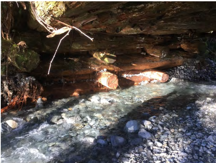
Right Bank Abutment when facing downstream
